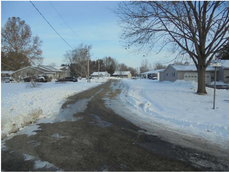
No further signage on Holcomb @ Kell on to Circle Dr.
